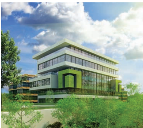
Office building - DN1A
